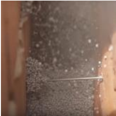
Wall cavity insulation
